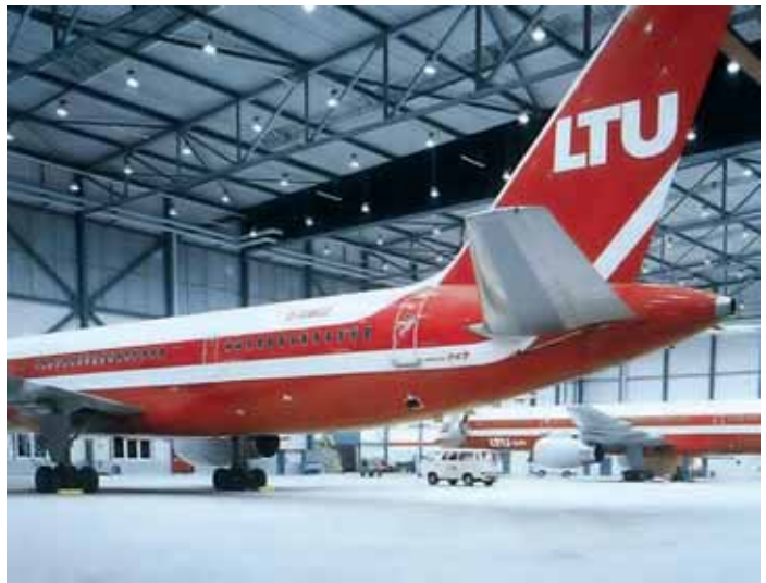
Fig. 4 Underfloor heating systems are used to heat maintenance hangars. (Source: Velta/Uponor)
