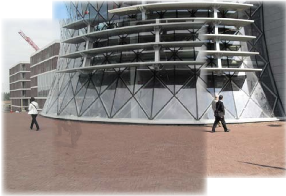
The “Gen Coel” Energy Center hosted the Conference, located in Heerlen, the Netherlands. The building features shading that tracks the sun.
