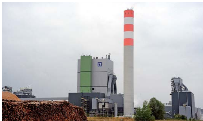
Lignin platform biorefinery for materials, power and heat from lignocellulosic crops or residues. Courtesy Zellstoff Stendal, Germany; and Task 42.
