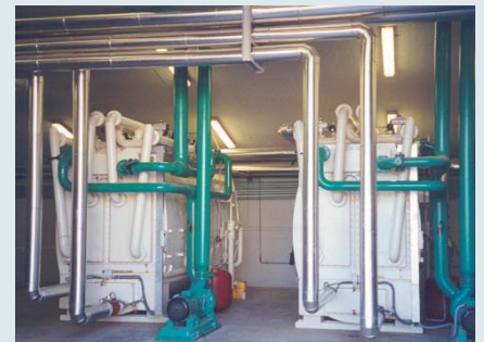
Figure 1: largest solar cooling site at present, Greece (site owner: SARANTIS S.A.): 2500m 2 collector area, 2x350 kW adsorption chillers (source: SOLE S.A. - design and installation)
