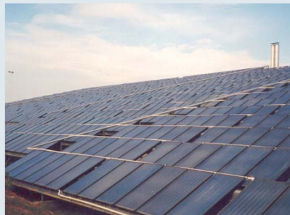
Figure 1: largest solar cooling site at present, Greece (site owner: SARANTIS S.A.): 2500m 2 collector area, 2x350 kW adsorption chillers (source: SOLE S.A. - design and installation)
