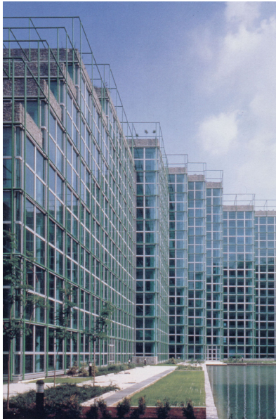
Figure 1 – V Palazzo SNAM (mechanically ventilated façade).
