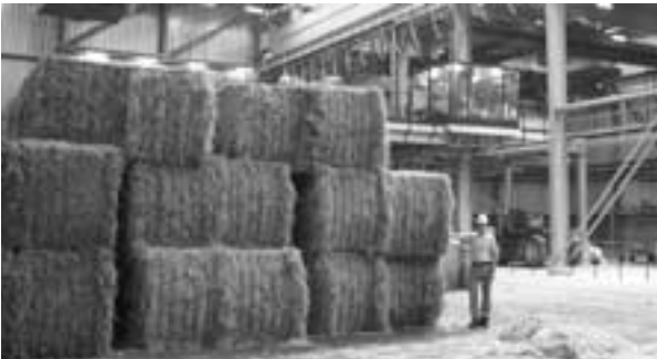
At full capacity, Avedøre 2's straw boiler burns 1200 bales per day. Each bale weighs 500kg. (Courtesy Thomas Scott Lund, Energi E2, Denmark)
