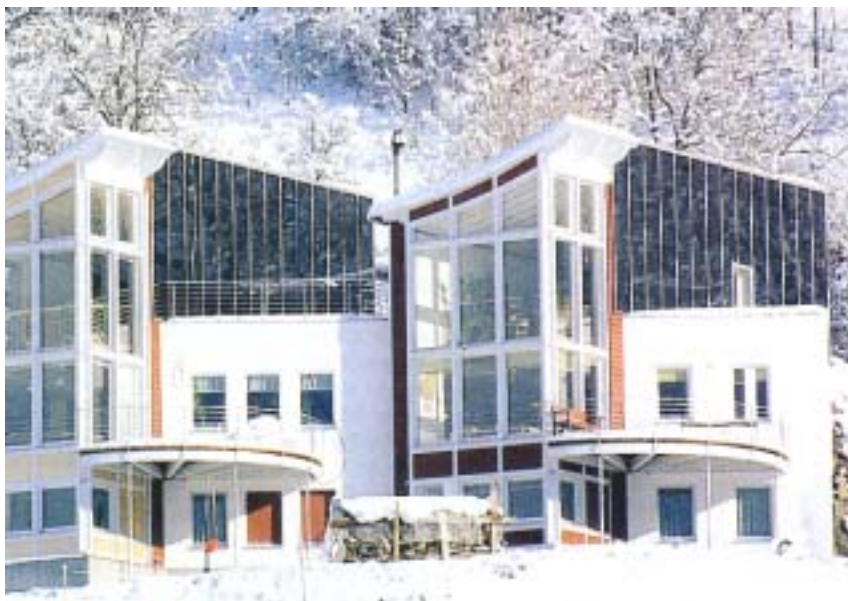
Figure 1: Buildings with large solar heat collectors for space heating and hot water preparation
