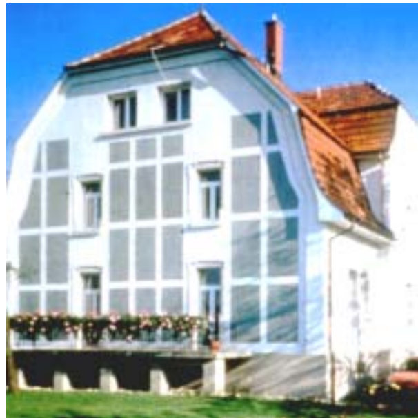
Figure 3: Retrofitted building with Transparent Insulation elements
