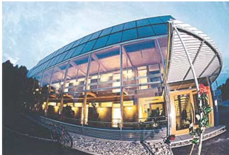
Figure 5: 60% of the space heating demand of this terraced houses are covered by solar energy (Source: AEE)
