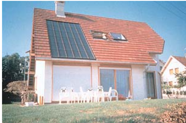
Figure 7: French house, equipped with a direct solar floor system (Source: Clipsol)
