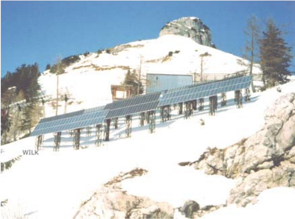
30 kW grid-connected PV-plant on the mountain Loser, Bad Aussee/Austria
