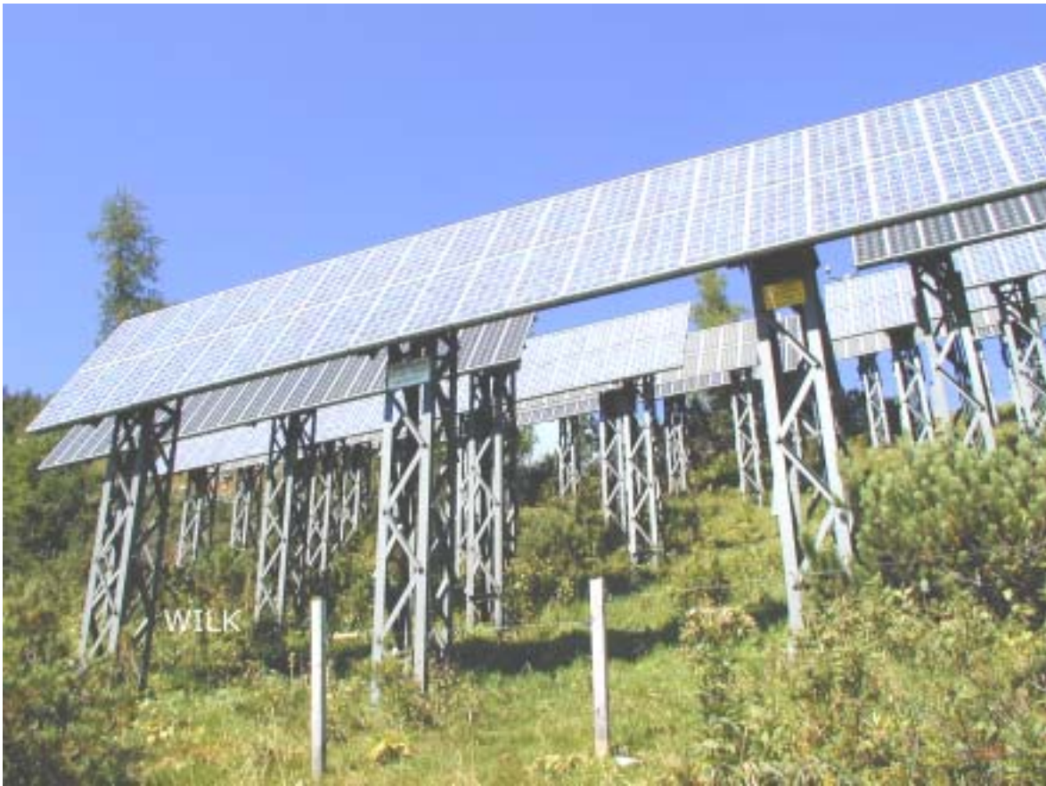
30 kW grid-connected PV-plant on the mountain Loser, Bad Aussee/Austria
