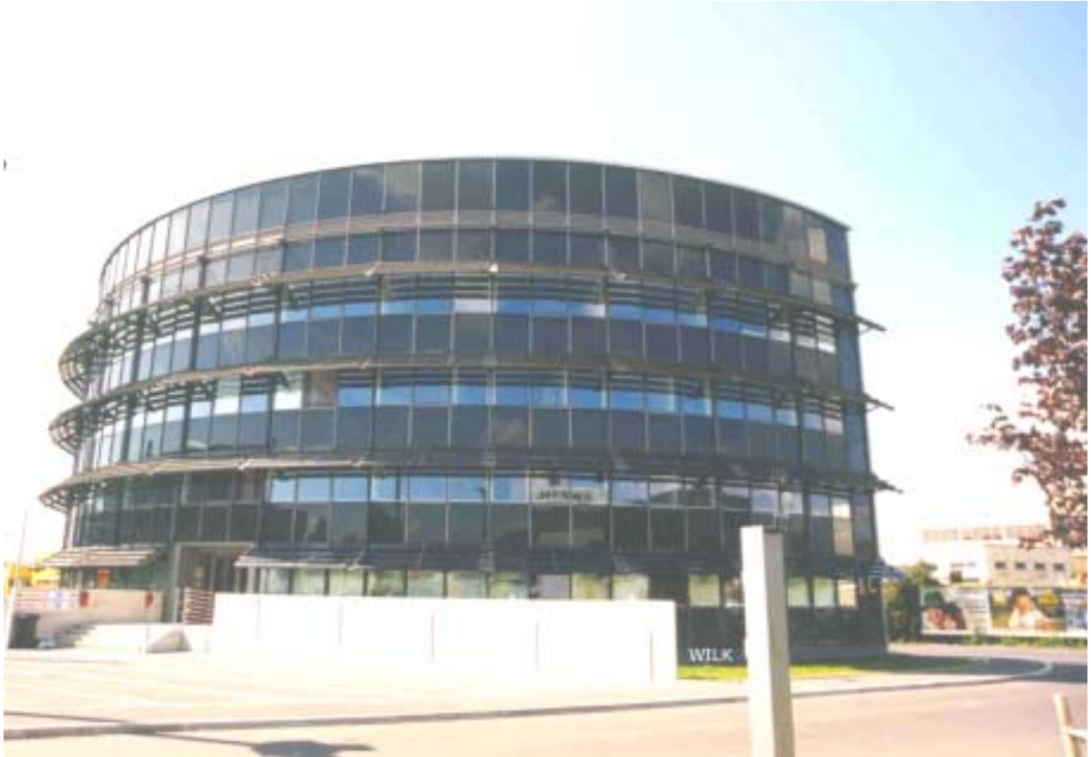
Façade-integrated 20 kW-PV-system in the office of SBL-Linz, Austria
