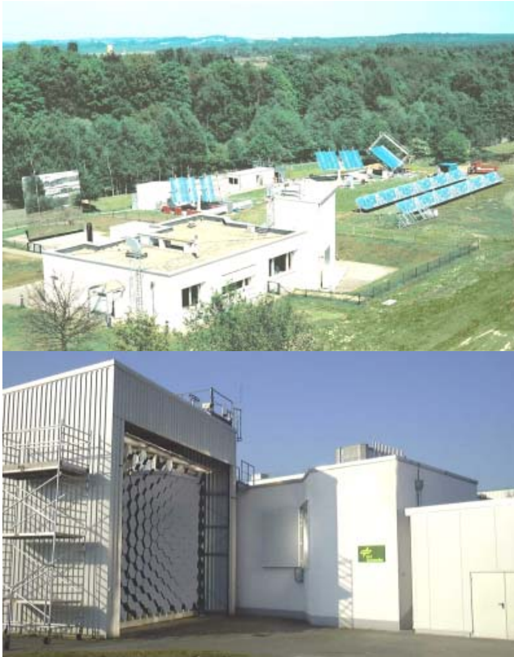
Fig. 3: Up: Areal view of the outdoor solar test facilities at the DLR in Köln-Porz, Germany. Foreground from left: laboratory building, concentrator building of the solar furnace, IST trough for solar process heat applications. Background from left: heliostat of the solar furnace, PROPHIS-plant for photochemistry, PAREX-plant for thermal components' tests, fix focus trough for thermal tests. Below: View of the concentrator, 147 spherical facets. One can see the opening to direct the light beam into the experimental room and the combined shutter / attenuator in a closed position on the right hand side.
