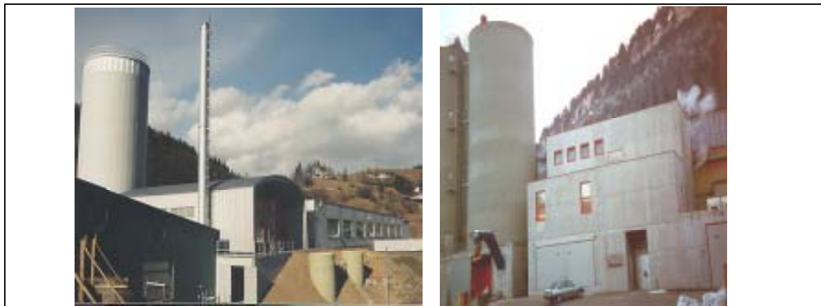
Fig. 5: Biomass district heat plant at Passail, Austria (left); Steam CHP plant at Reutte, Austria (right)
