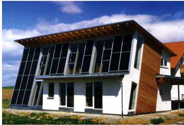
Fig. 1: Solar Combisystem with facade-integrated collector array (Source: Wagner & Co, Germany)
