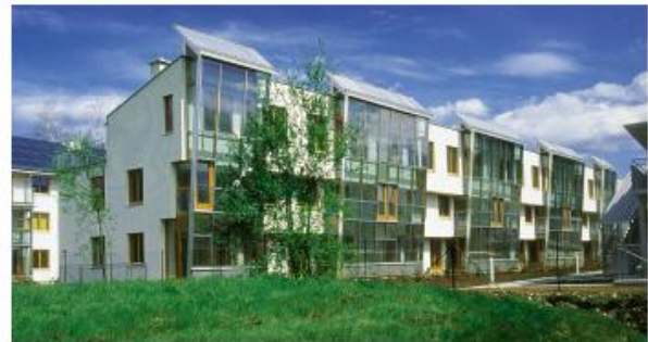
Fig. 8: Solar supported heating system for housing estate
