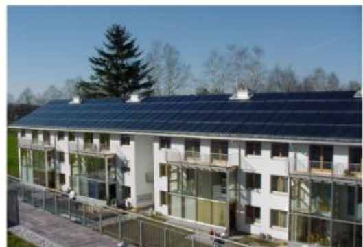
Fig. 3: Solar hot water system for multi-family housing
