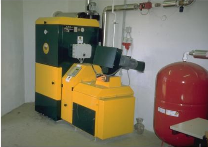
Fig. 8: Biomass heating for housing: pellets boilers
