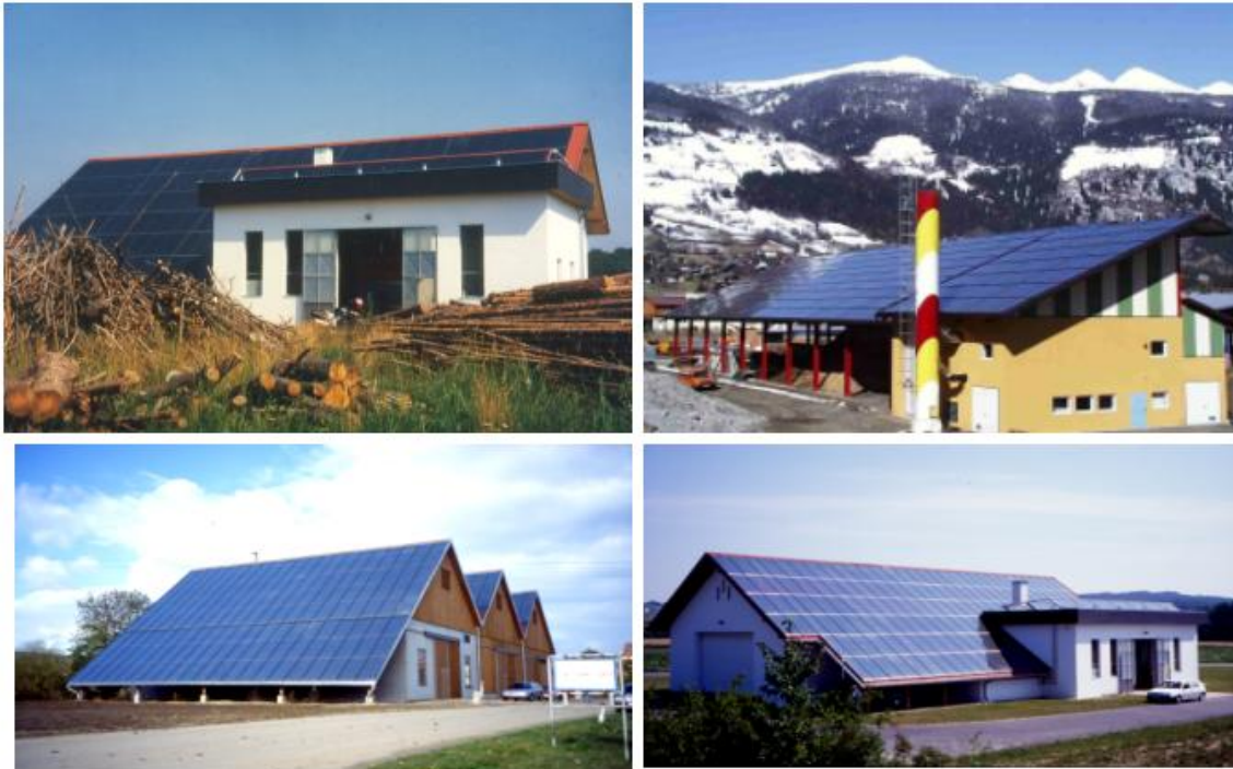
Fig. 6c: Solar hot water system for biomass district heating
