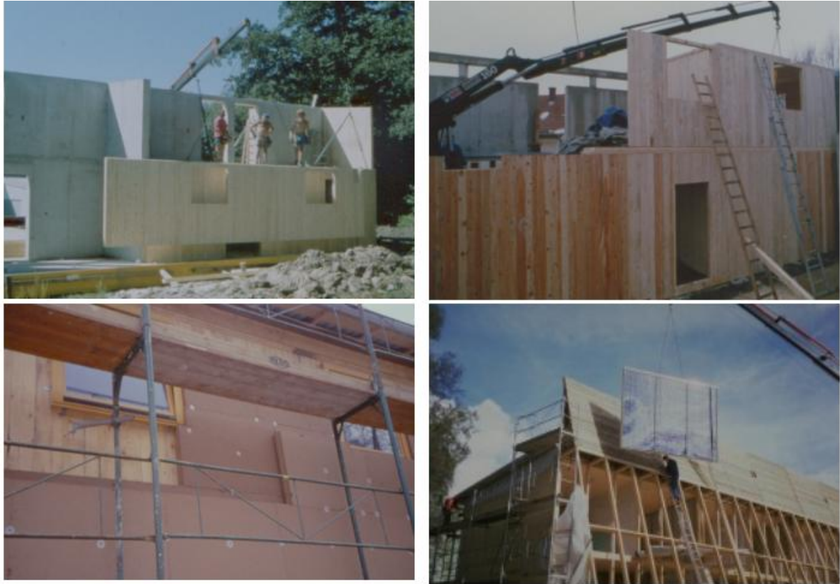
Fig. 5: Building construction phase
