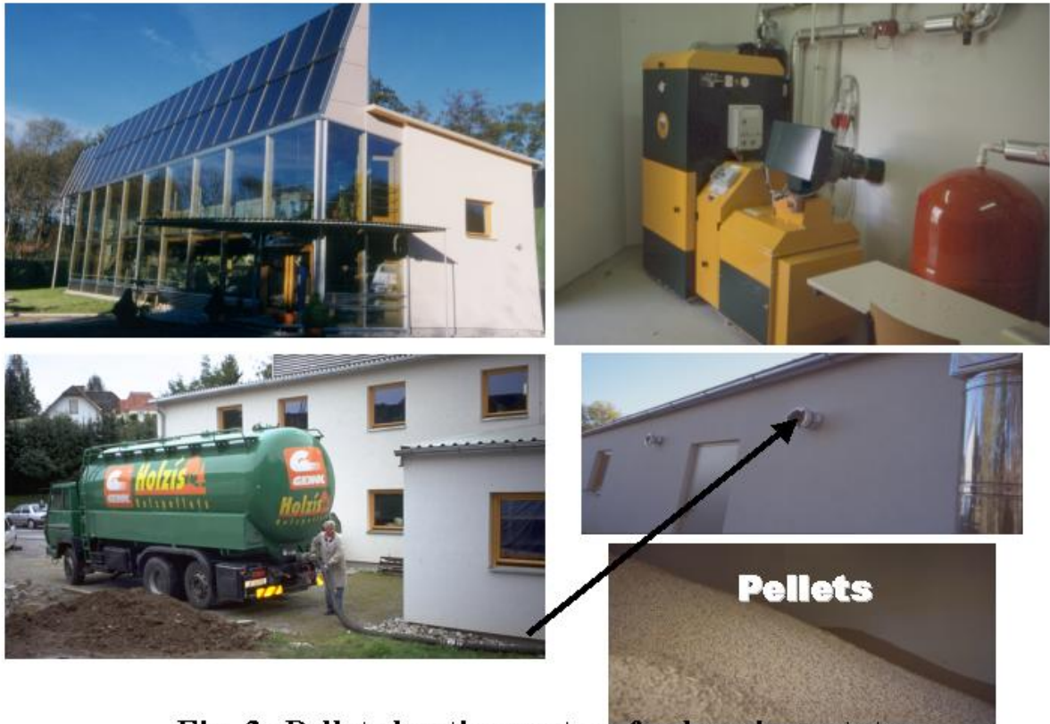
Fig. 3: Pellets heating system for housing estates
