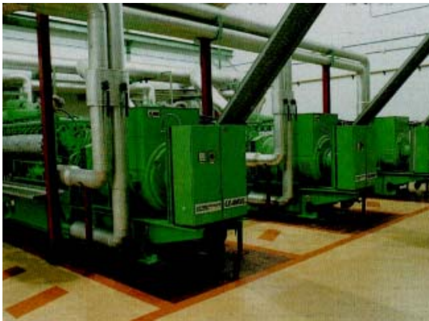
Figure 24: Block CHP plant with modular construction
