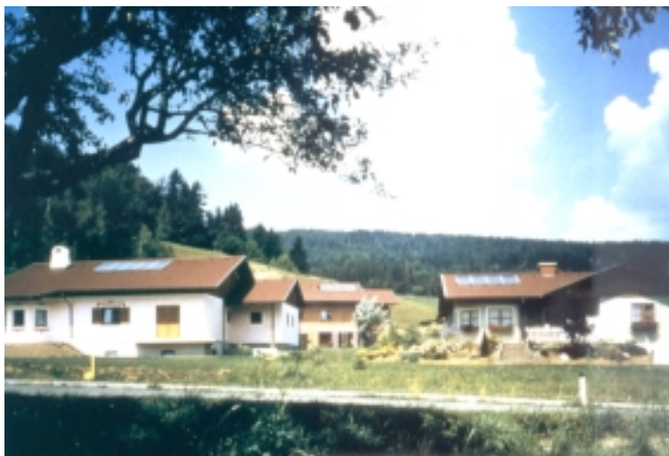
Figure 15a. Single family houses with solar hot water systems
