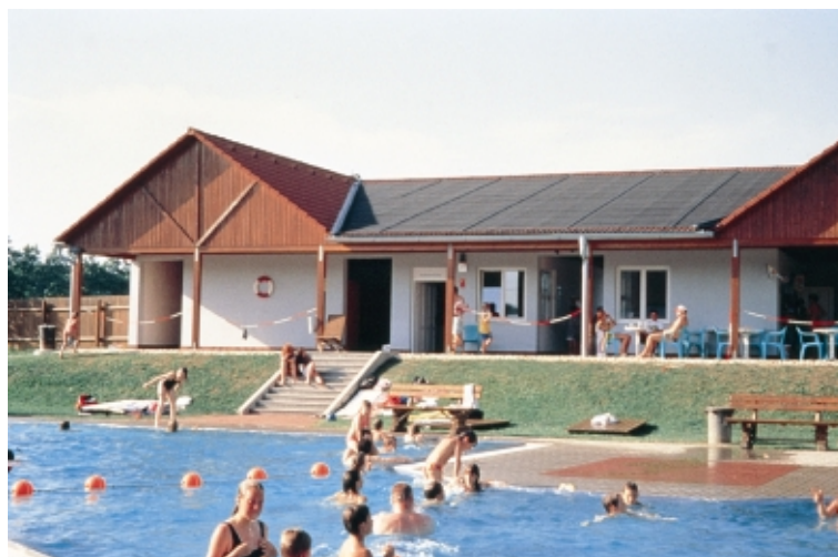
Figure 14a: Solar plant for pool heating
